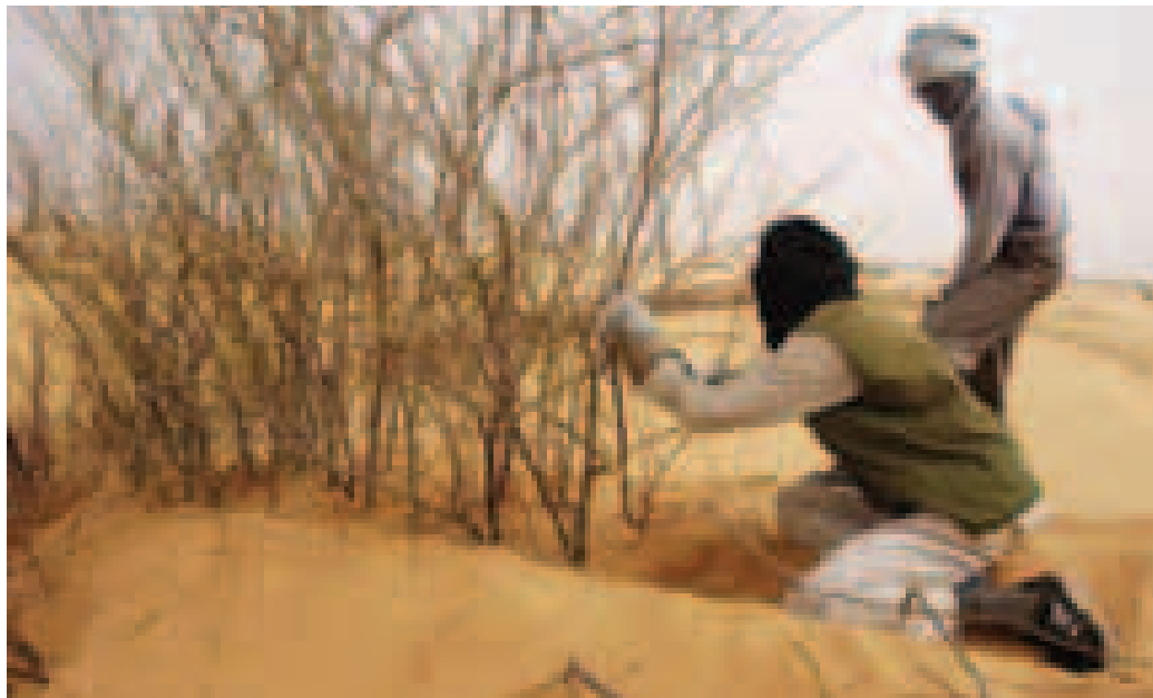
Installing a palisade or fence
