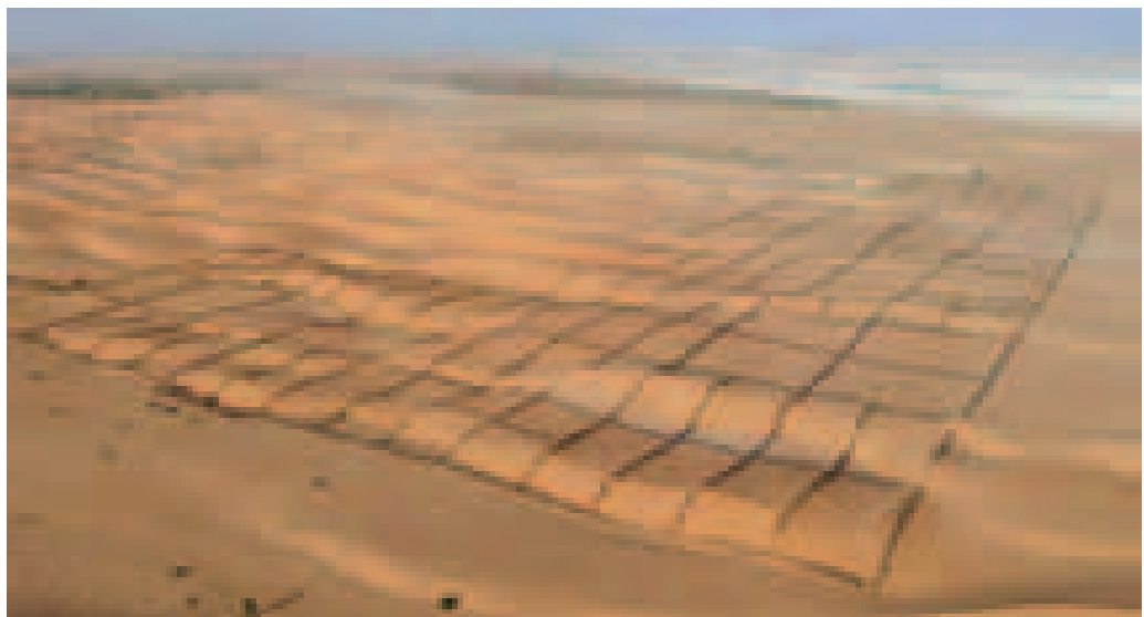
General view of a mechanically stabilized area
