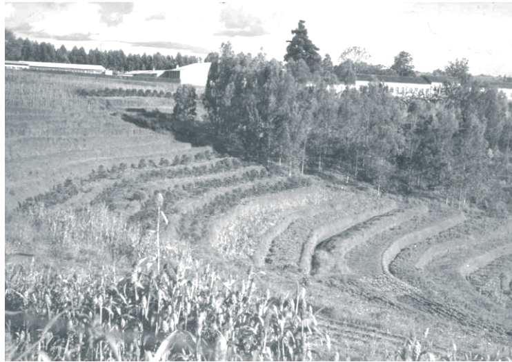
Figure 10. Bench terracing is in use in Rwanda since 1976. Never there have been reports on failures. The benches are slightly slope inward inclined and a 100 % infiltration is realised. This is absolutely necessary to prevent destruction of the whole slope by gullyng.
