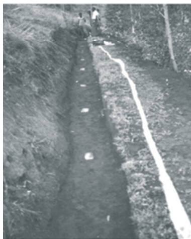
Figure 5. collector trench at Butare
