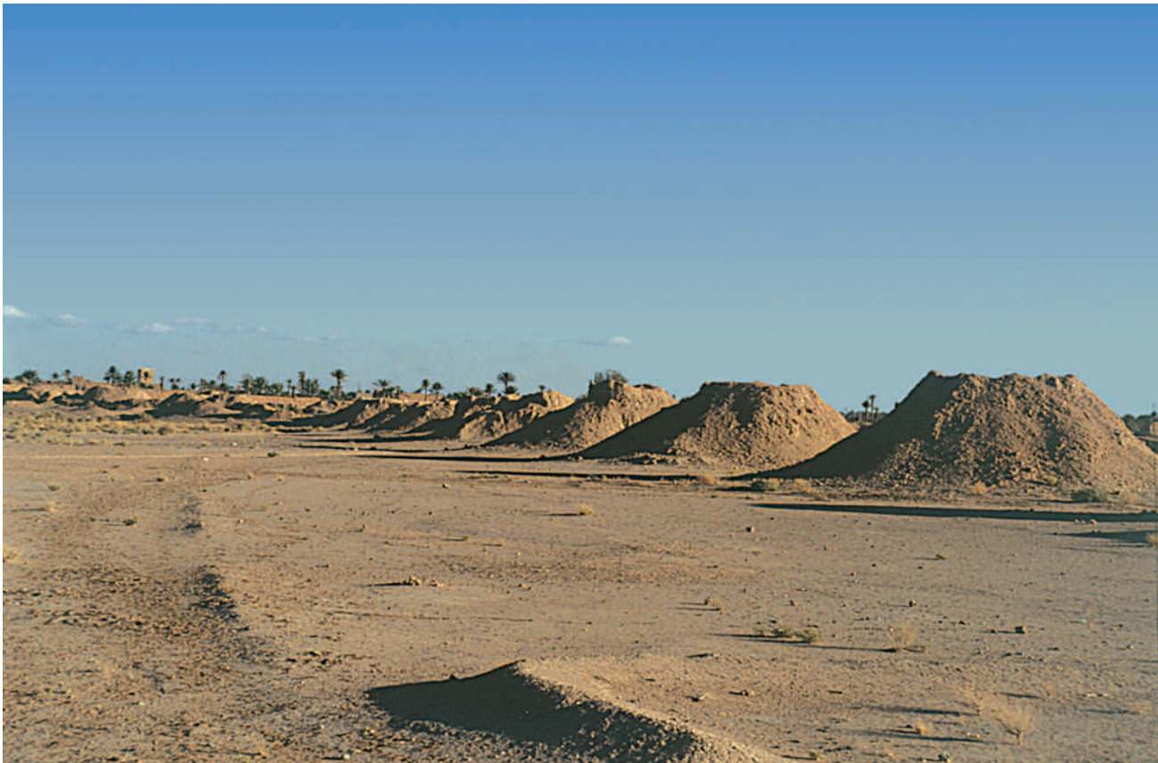
208-09. Morocco. Above, vegetable fibre barriers to stop soil erosion and provide protection from sandstorms. Below, restoration of the drainage tunnels and the air shafts. The Moroccan foggara system allowed the building of the complex urban layout of the medieval capitals. When the foggaras were abandoned entire towns completely disappeared.
