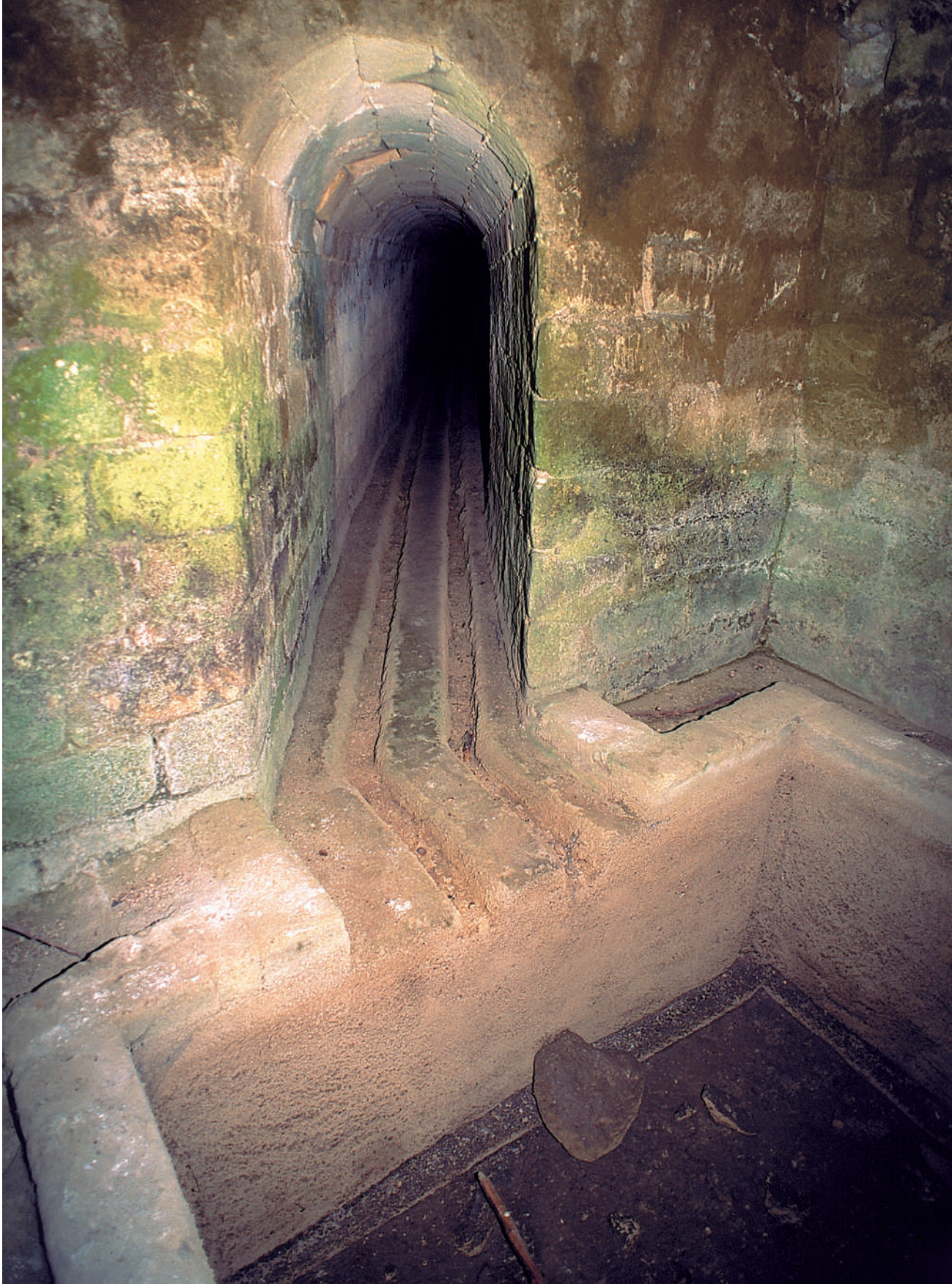
173. Gravina in Puglia. The underground tunnel of the water system, very similar to the Saharan drainage tunnels, supplies the fountains in the historical centre of the town, situated on the opposite side of the canyon, by means of an aqueduct-bridge which is, in its turn, supplied with water tapped on the hill of Botromagno.
