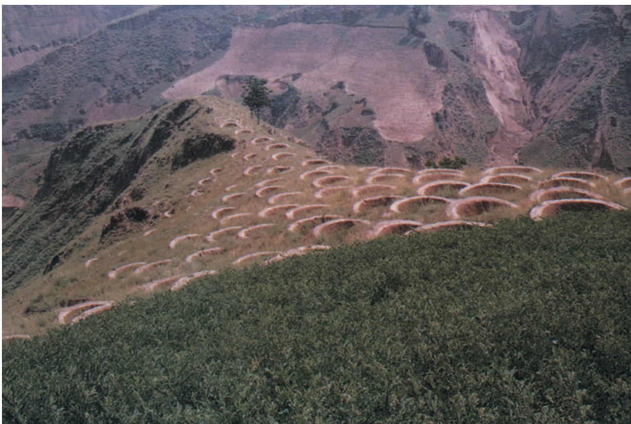
194-195. China, soil protection system on a large scale. Above, vegetable fibre barriers to stop the sand. Below, dry stone lunettes for the creation of soil and the protection of the slopes.
