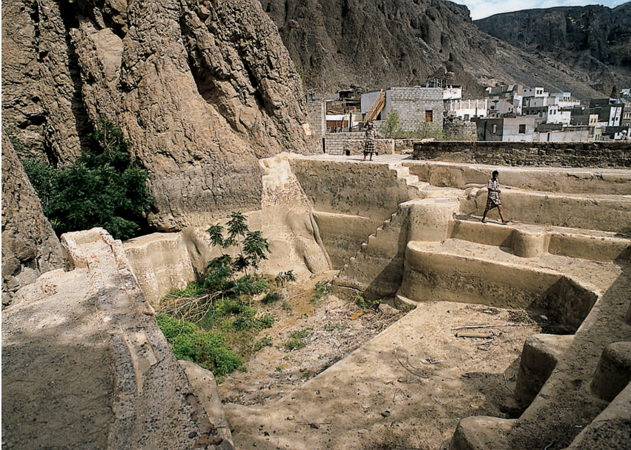
61. Detail of the cisterns of Aden made watertight by means of the traditional plaster that is particularly water-resistant.
