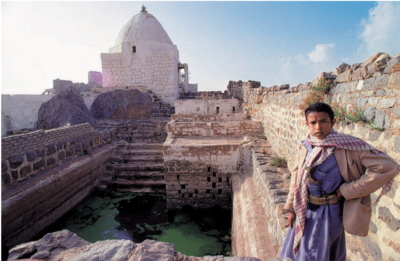
135-136. In Yemen mausoleums and holy places are almost always related to water harvesting. Fig. 135, the Hadramaut valley: the sanctuary above channels the runoff along the slope into the room of ablutions and prayer below. Fig. 136, northern Yemen: the rainfalls collected in the courtyard for prayer fill up the open-air cistern.
