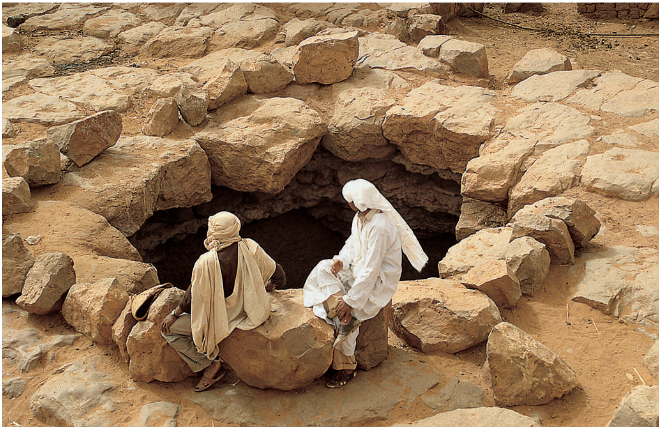
105-106. The heaps of stone on the surface, resulting from the excavation wastes of the vertical air shafts, show the underground layout of the foggara. Below, air shaft of the drainage tunnel which opens beneath the built-up area into large cavities for ablutions and cooling.
