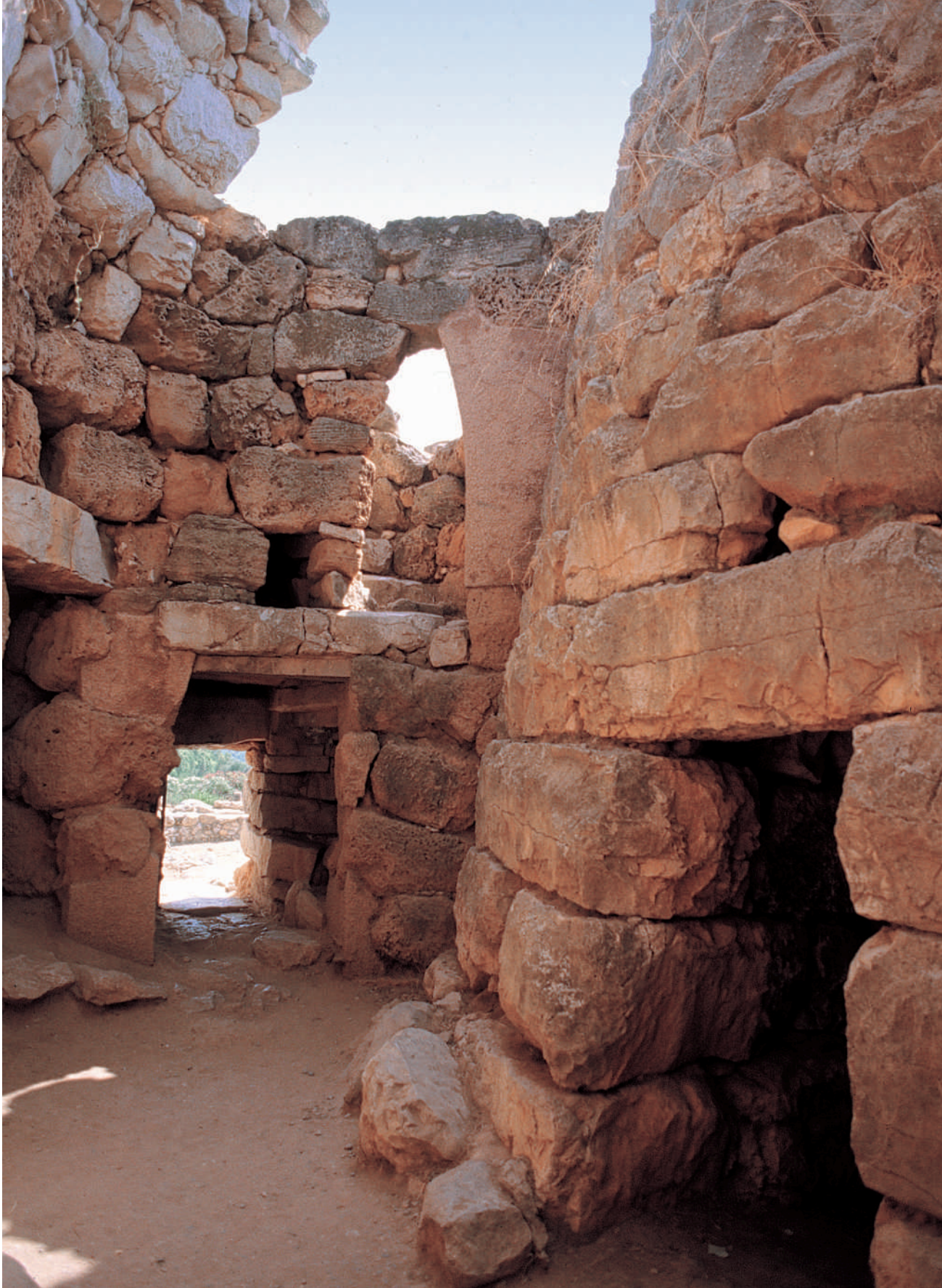
64. Nuraghi of Palmavera (Sassari). The massive double wall circle has the practical purpose of condensing humidity and preserving water in the underground hydraulic devices, like the principle on which the southern Arabian mahfid are based.
