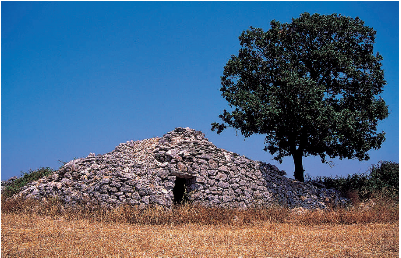
86-87. Above, Cleopatra Selene's mausoleum (Algeria). The construction derives from the megalithic barrows of the Numidian tradition called medracen . Of the same typology are the Apulian barrows and specchie (see figure below), whose masonry enables the moisture absorbed by the tree roots to be conserved in the soil.
