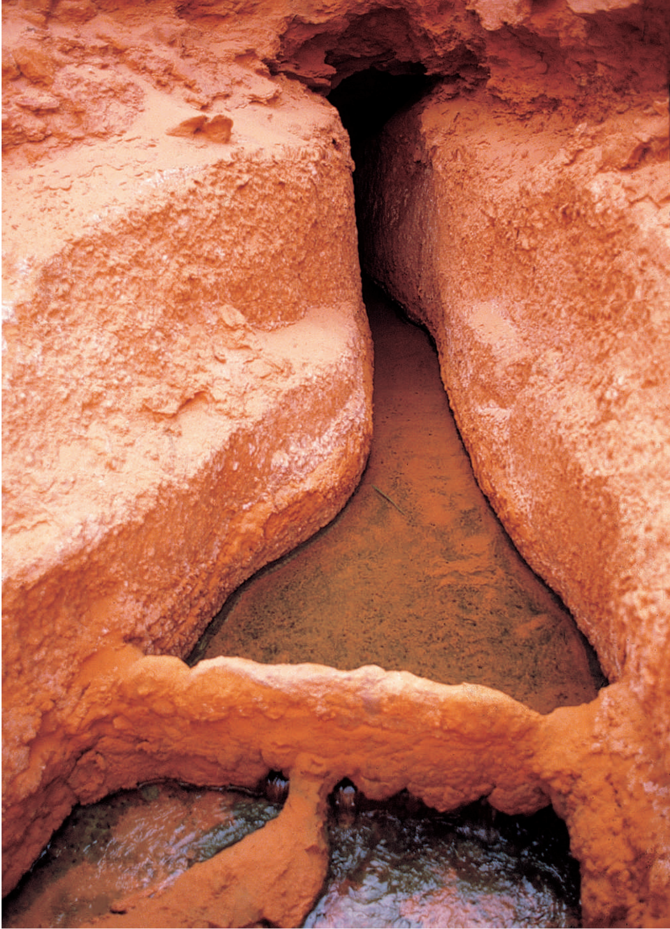
104. Oasis of Timimoun (Algerian Sahara). The water sharing system at the surface outlet of the foggara.
