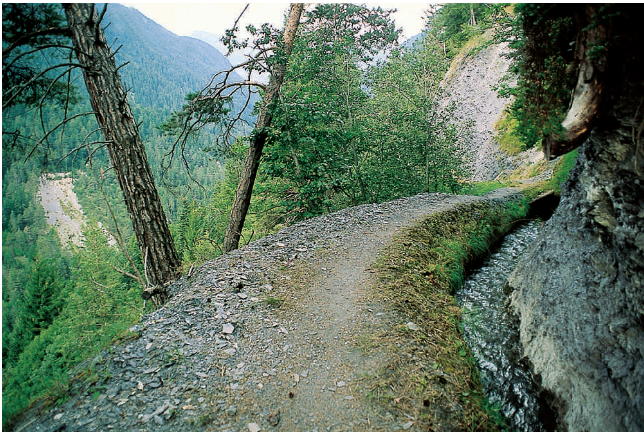
178-79. Valais (Switzerland). Channels called bisse collect water coming from the glaciers melting along the long pathways carved out of the sides of the mountains and use this water to irrigate the otherwise completely arid valleys.
