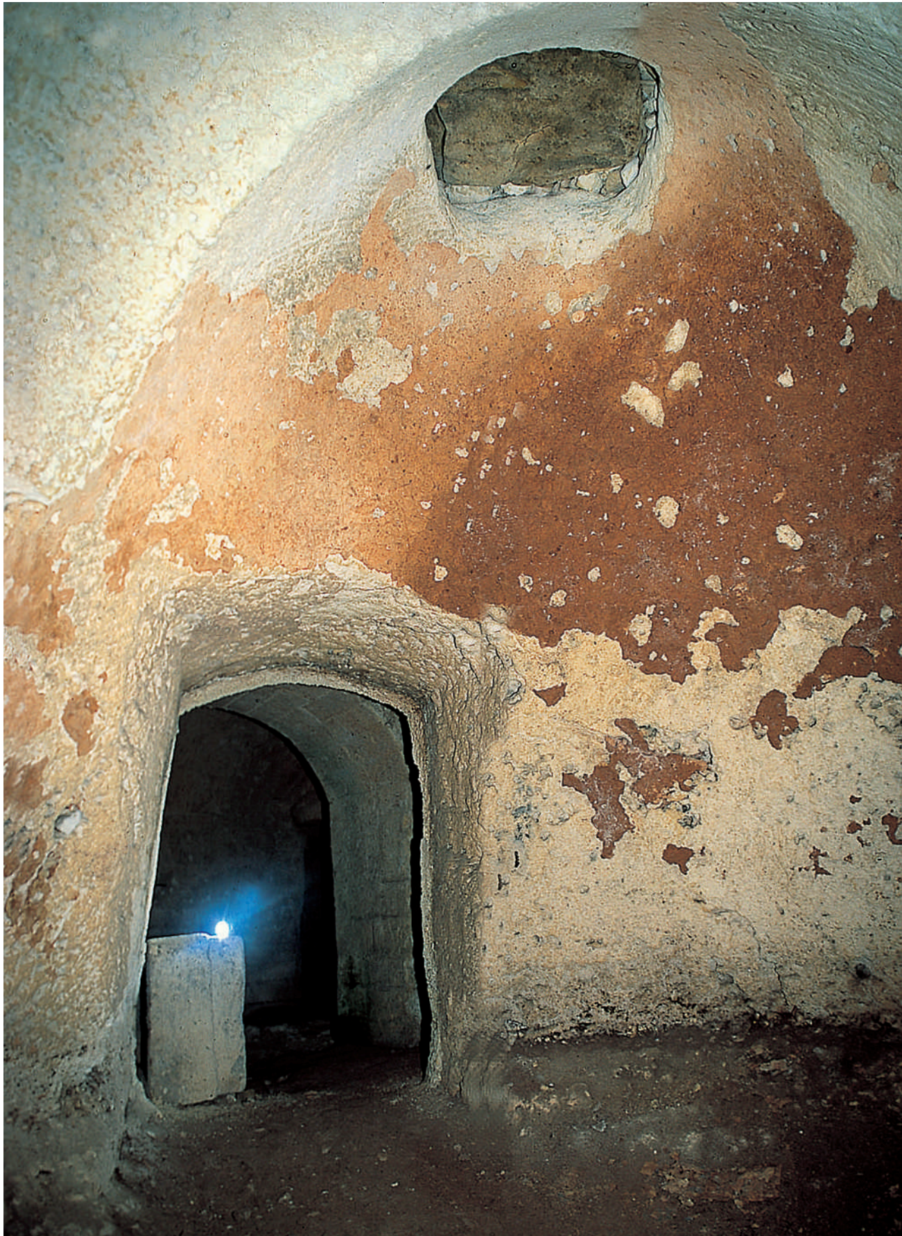
81. Bell-shaped cistern in the Sasso Barisano of Matera subsequently reused as an underground room. Note the orifice at the top for the water, and the watertight plaster of a reddish colour due to the pottery shards used in its making.
