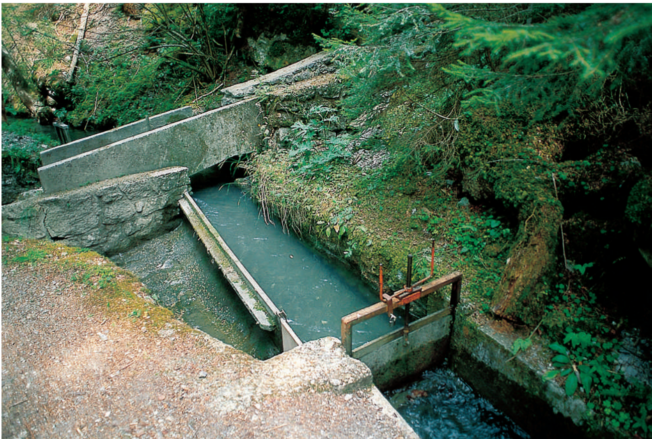
210-11. Valais (Switzerland). The practice of the channels ( bisse ) is still used and supported by community interests and rules. Above, diversion of the bisse by means of a traditional irrigation device. Below, sluice gate and water sharing system.
