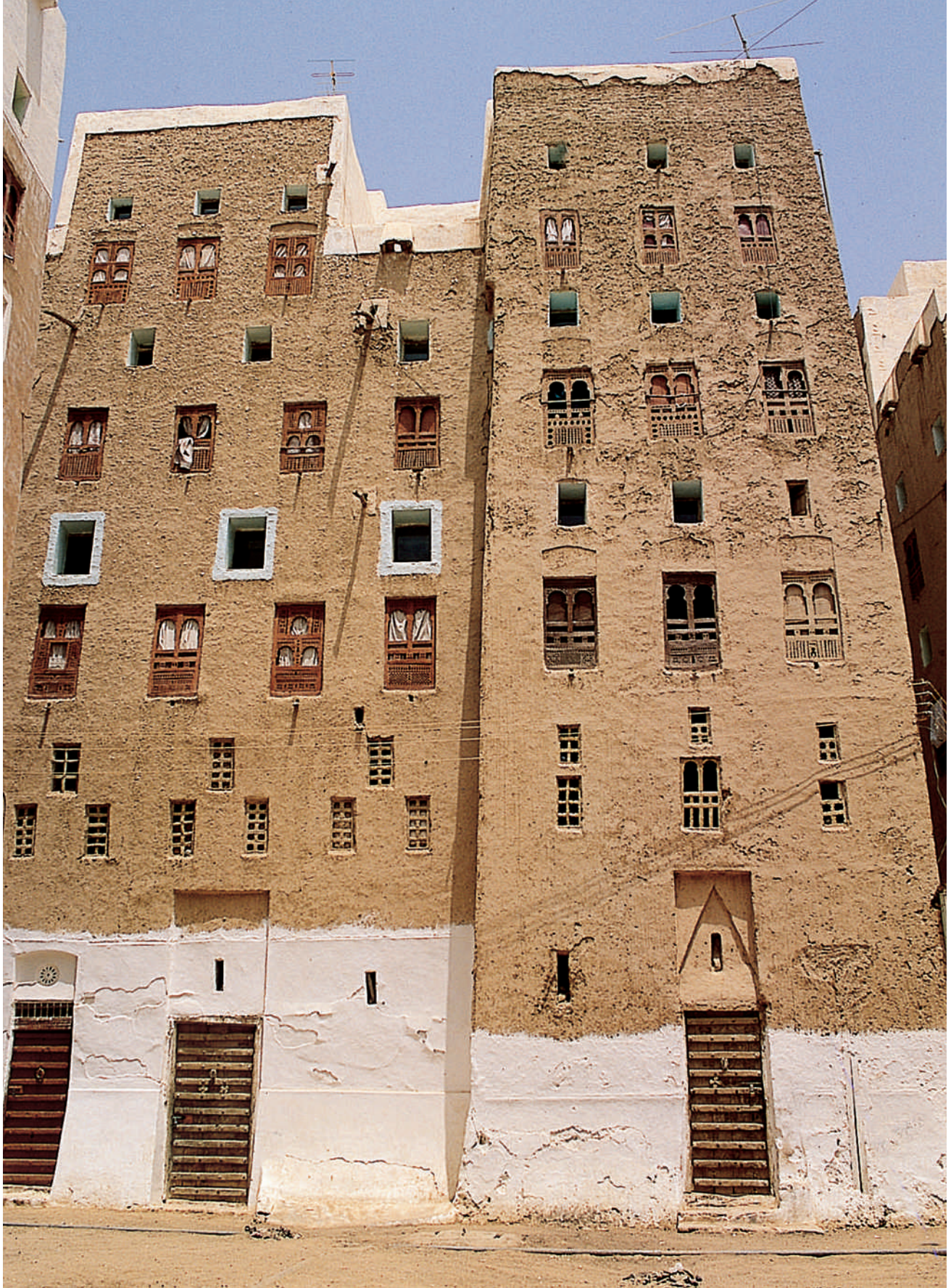
134. The dwellings of Shibam are tall tower-houses made of raw earth. Each house is inhabited by a single family which is able to build the massive construction thanks to the low cost of the material.
