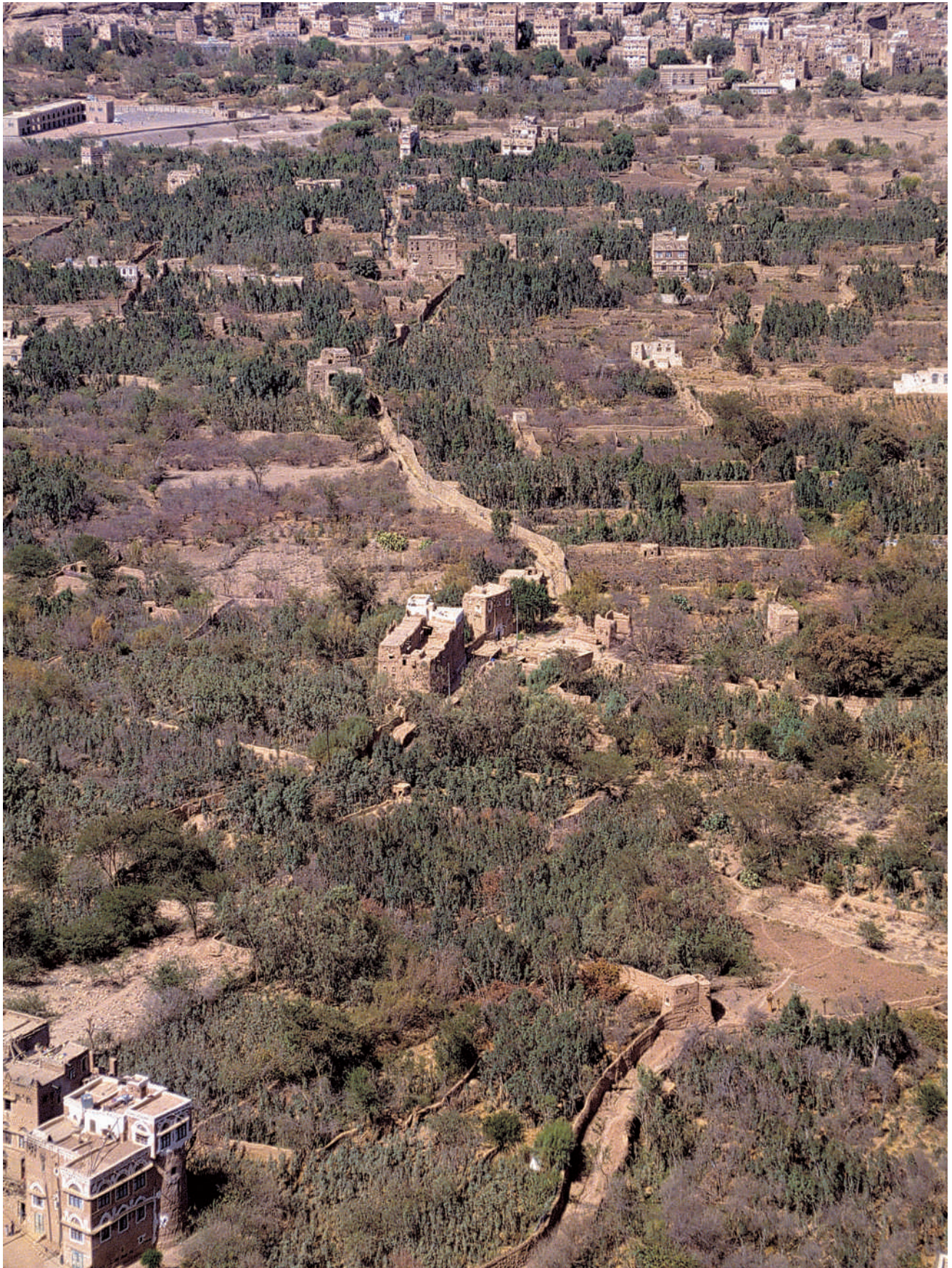
128. Wadi Dhahr (Yemen). The landscape of roads, gardens and cultivations created thanks to the water distribution technique of the torrent-streets. The water intakes open into the gardens situated between the walls of the narrow streets. The whole system works by gravity and determines a rigorous organization which fully functions only when of the sporadic floods occur and the pathways turn into watercourses.
