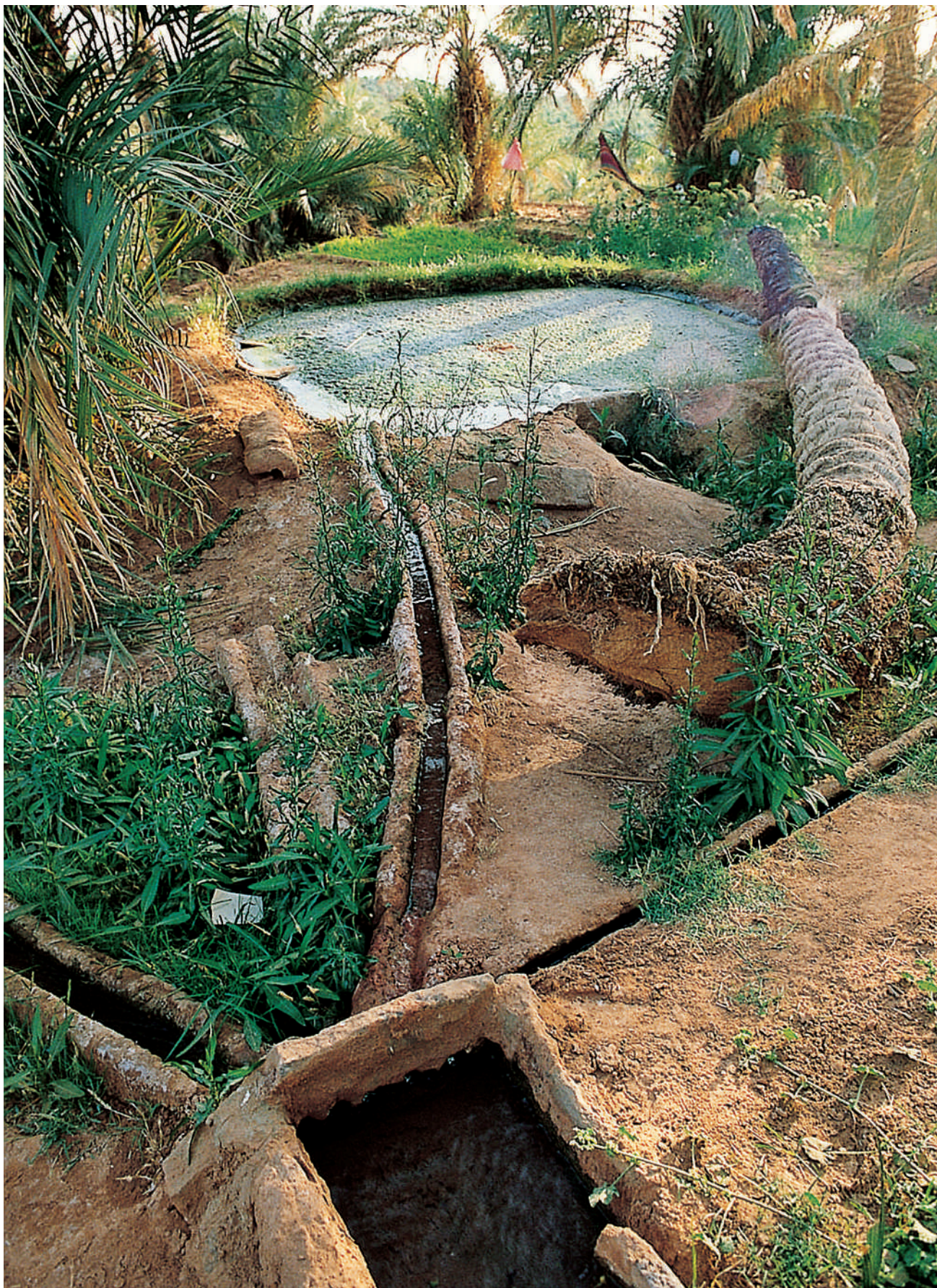
112. Water is distributed to each owner by a series of channels on the surface and is temporarily collected in small basins called majen. The shade of the palm trees and the formation of algae on the water surface obstruct evaporation.
