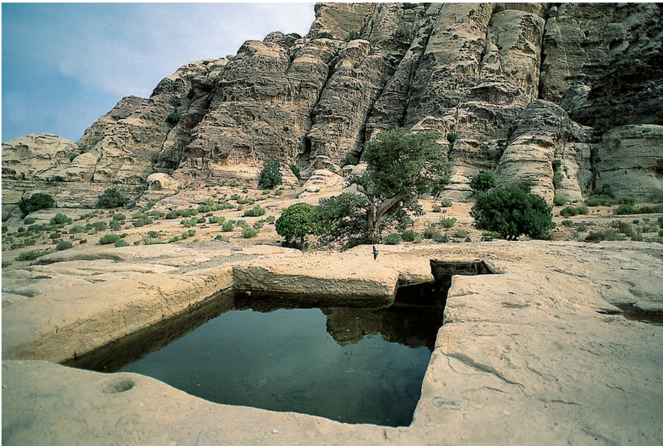
154-155. The upper part of Petra is the holy summit where the first rains and the night dew are harvested in a double circle pool. Later water is conveyed downstream to the cisterns (photo below).
