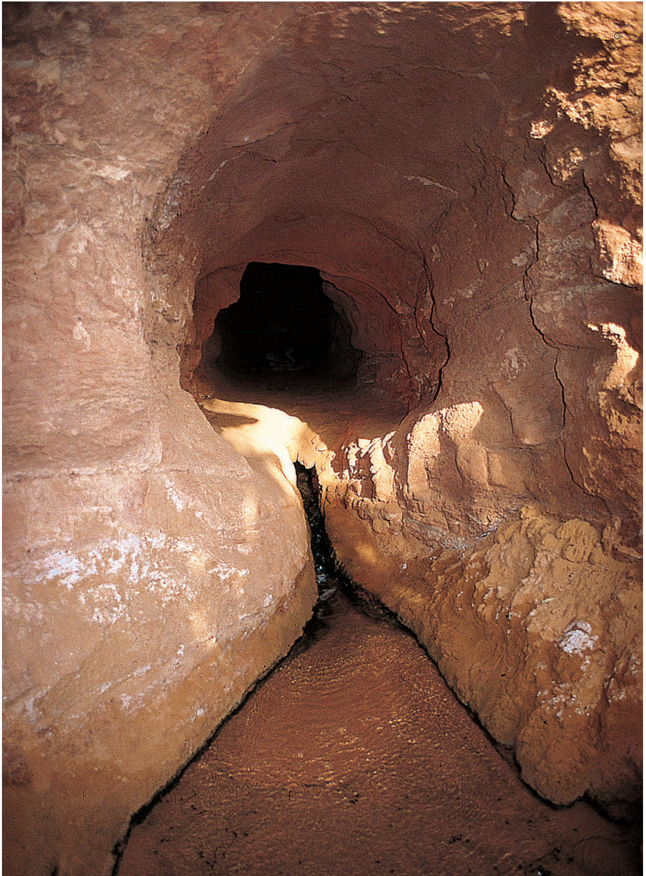
103. Oasis of Timimoun (Algerian Sahara), the interior of the drainage tunnel called foggara. The tunnel is dug out of the limestone rock and thanks to its linear development it is able to catch the quantity of water contained in the porous ground.
