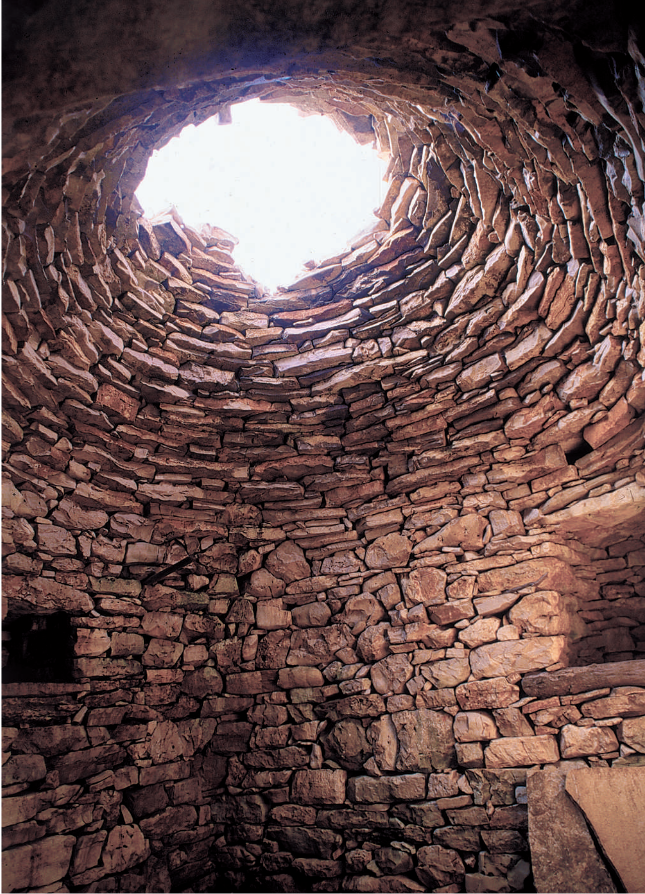
85. The interior of a trullo. Like the tholos, the covering of the trullo is a false dome which does not need a keystone on the top to support itself.
