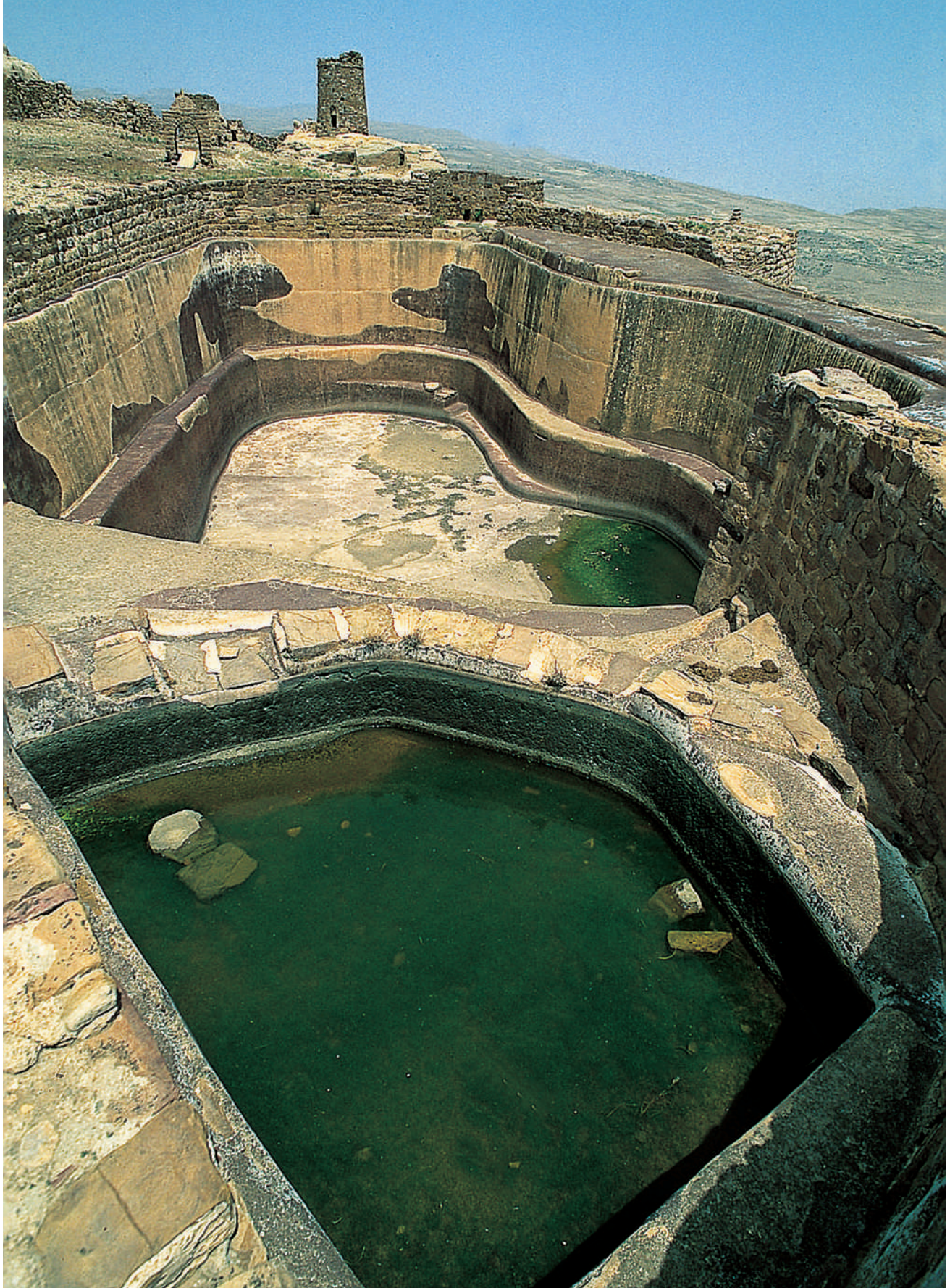
73. The large reservoirs for water conservation on the acropolis of Thula (Yemen) had sufficient dimensions to supply water to the fields and the surrounding houses and to withstand sieges.
