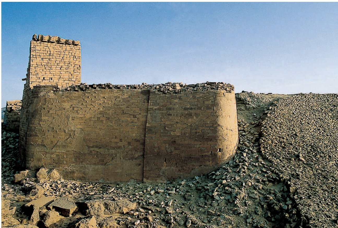
62-63. The southern and northern sluice-gates of the Marib dam (Yemen). It was a complex sharing system of the water intercepted by a dam which spread out perpendicular to wadi Dhana between the two sluices.
