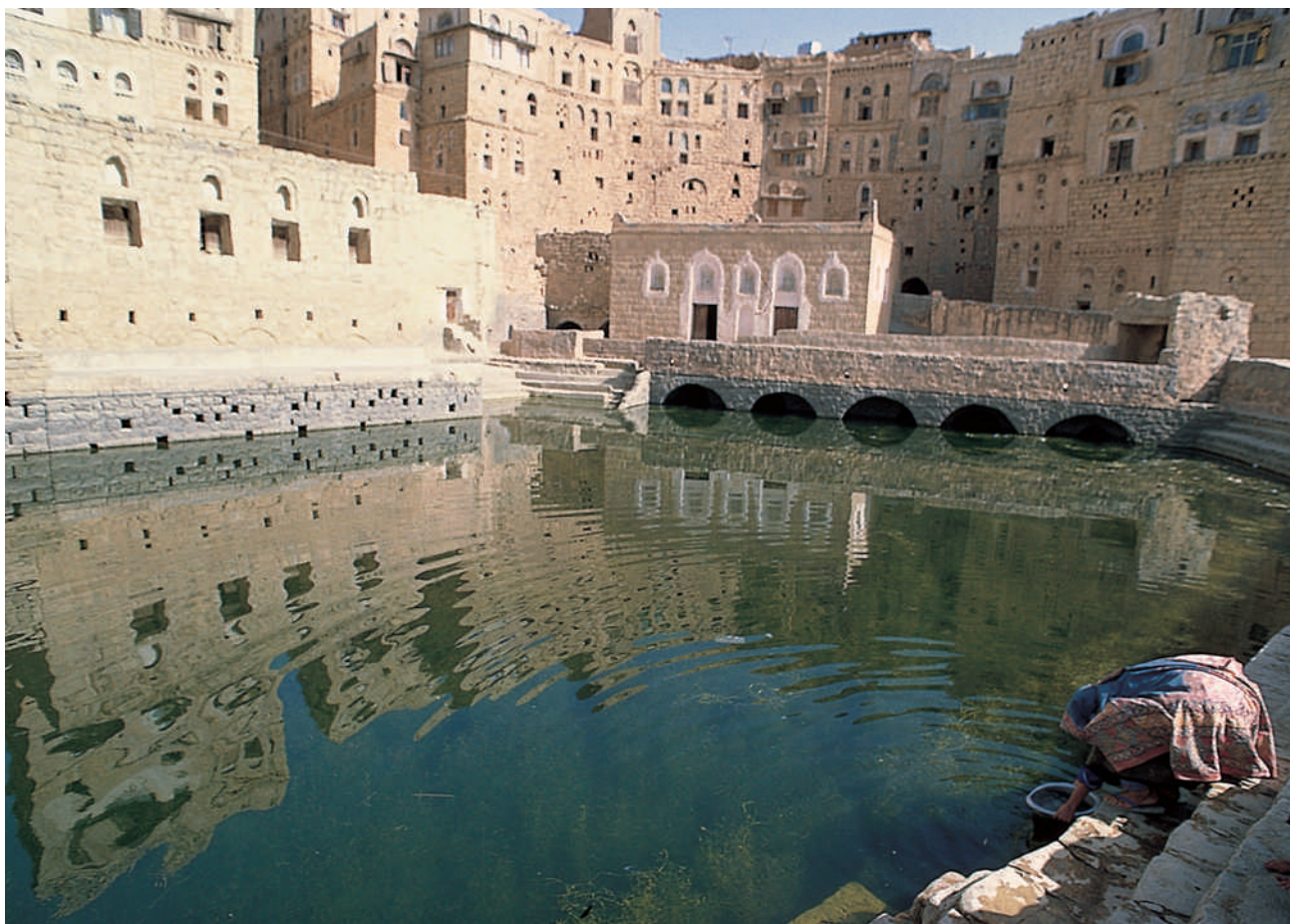
72. Hababa (Yemen). The town surrounds the large cistern-basin where the water coming from the terraces of the buildings is collected. The little building at the water's edge is a mosque with pools inside supplied with water by the big arches.
