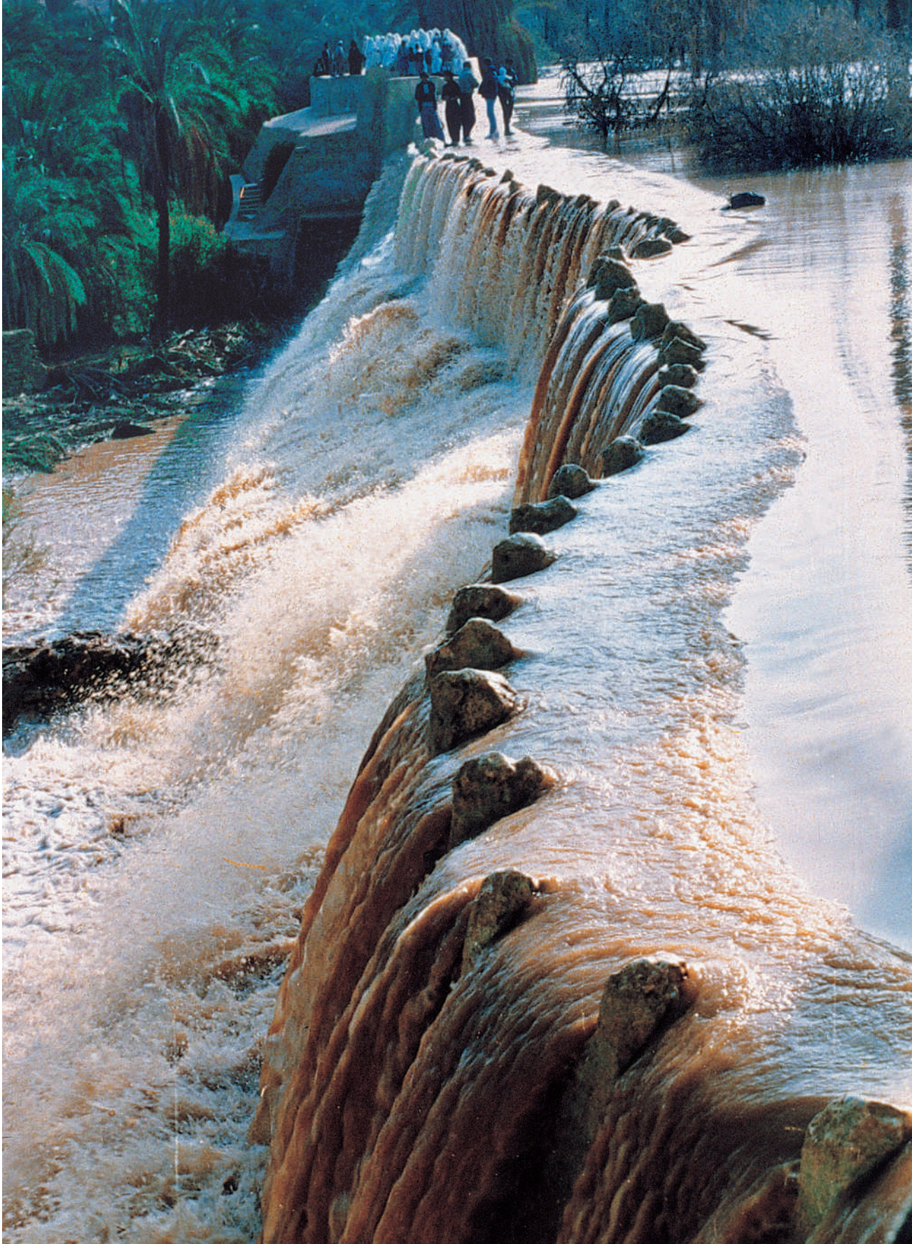
125. The dam of Beni Isguen in one of its sporadic moments of flood that even occur every ten years, when the water intakes channel the flows towards the single parts of the palm-grove and replenish the water table
