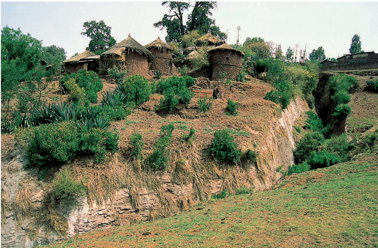
43-44. Village on the Ethiopian highland. Above, the general view shows the elliptic ditch like that of the Neolithic villages (see fig. 33). Below, detail of the ditch whose multipurpose function still now enables the built-up area to be kept dry and drained, creating a water reservoir and a sewage collection system for soil fertilisation.
