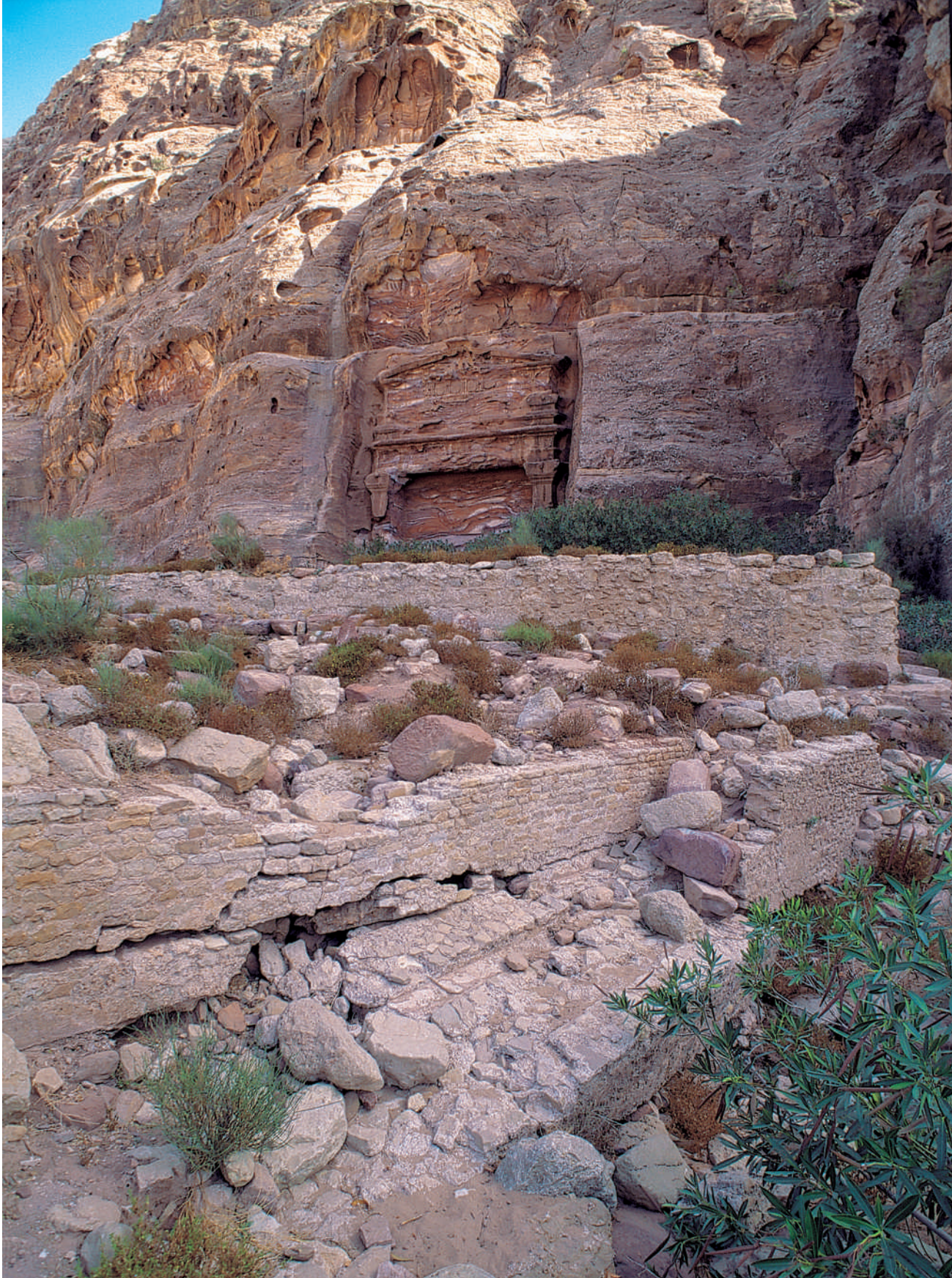
76. In Petra (Jordan) the stone terracing systems called khaur , typical of the Nabatean agriculture used in the Negev desert, are still visible. In rural environments, they are mere semi-circular terracing systems which retain the soil, whereas in urban areas they are more complex building systems. Some examples of these systems made with carbon layers to filter water and make it fit for drinking have been discovered.
