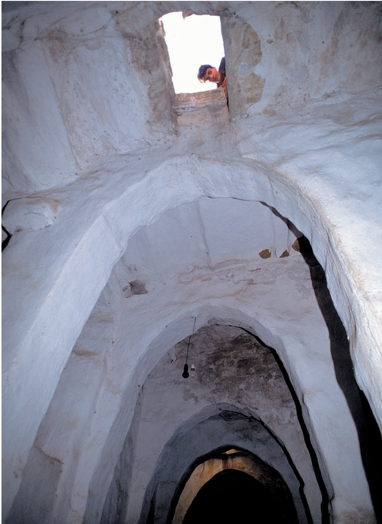
137. Yemen, underground cavities used for ablutions. All mosques always have hypogeal rooms which gather water. They are often devices which existed before and were built for the Sabeian temples.
