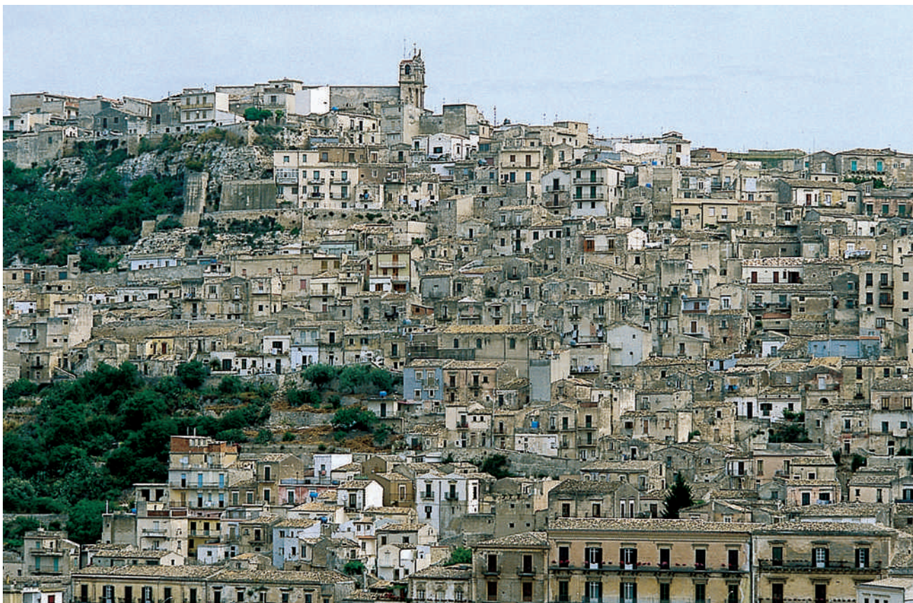
162-63. The old centres of the Hyblaeen region (Sicily). Above, Scicli and the built façades overlapping the network of underground structures. Below, Modica organised in concentric circles along the slope. The similarities with the Sassi of Matera and the ecosystems of the gravine are evident because of their common origin in the hydro-agricultural layout.
