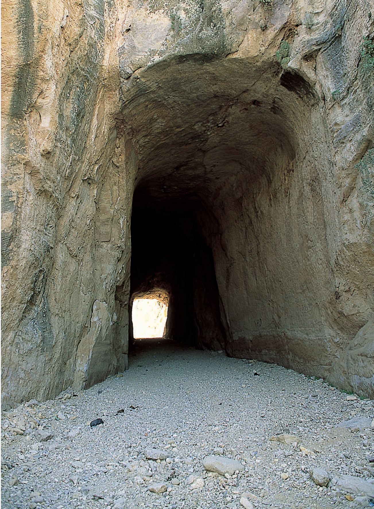
150. Petra, a tunnel excavated by the Nabateans to deviate flood water from their natural water course across the canyon at the entrance of the town, called Siq.
