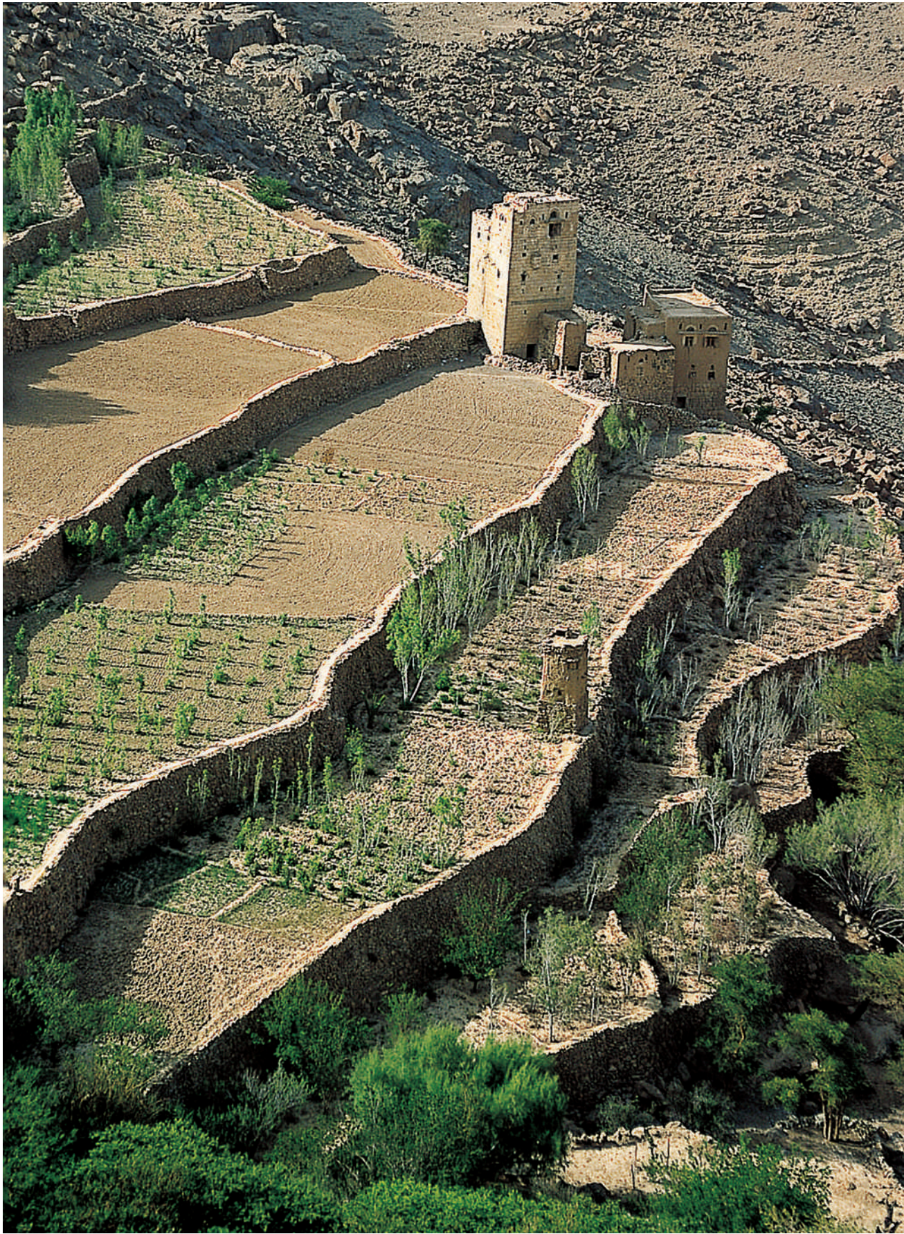
138. Yemen, terracing system for the protection and cultivation of the slope. The water intakes deviate the flows from their natural course and direct them along the walls on the terraces. Towers and stone buildings are placed to defend the cultivations.
