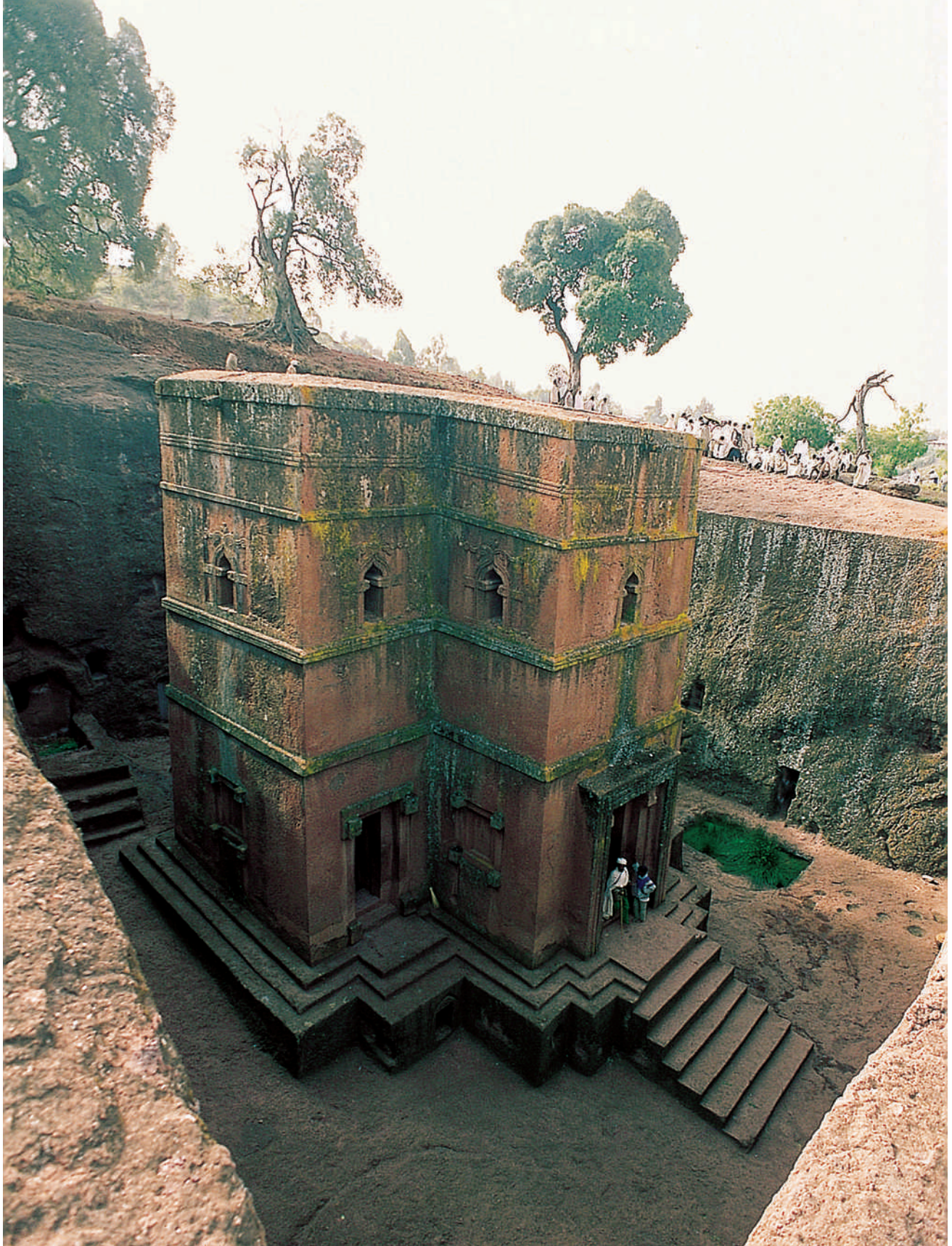
40. Lalibela (Ethiopia), monolithic hypogeal church of Biet Ghiorgis (12th century AD). The roof of the church is level with the surrounding plain. The building technique of the monolithic hypogeal structures consists of a courtyard dug in the plain and a block of rock left in the middle which is worked into architectural forms. The windows are hollowed out and through them internal storeys with colonnades, capitals and architectural orders are excavated. The result has the appearance of built architecture which is actually dug out of a monolith.
