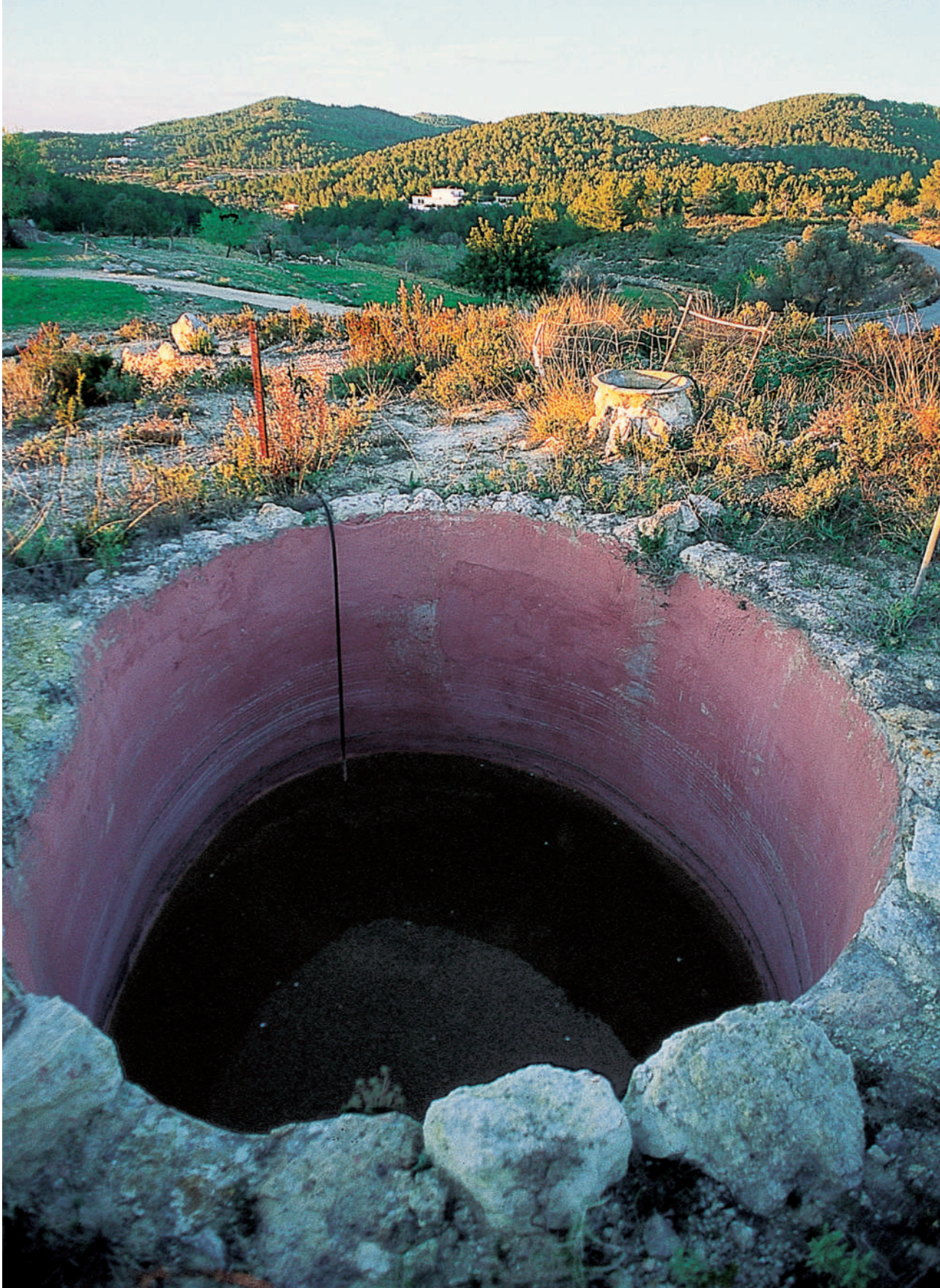
130. Ibiza (Spain), cistern and cistern-jar. The system of the cistern-jars, underground water reservoirs, is spread throughout the islands and along the arid Mediterranean coasts, providing a reserve known to travellers who used it during their journeys.
