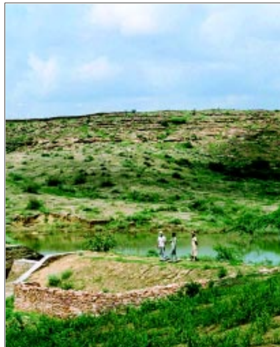
Community water dam
