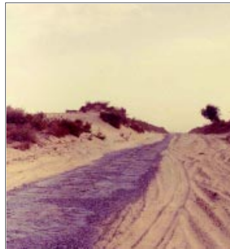
Encroachment of moving sand onto roads
