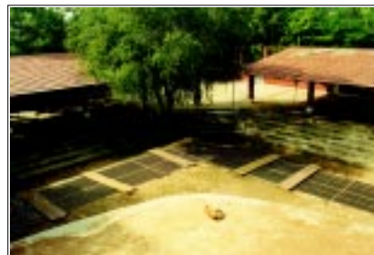
Underground water storage at the SWRC compound
