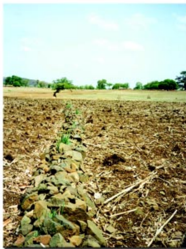
Vegetation and stones are used to build anti-erosion dykes
