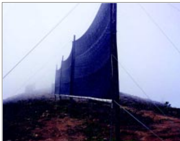
Fog-trapping nets capture moisture from the air
