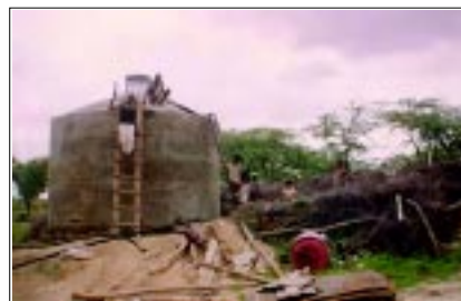
Constructing a water storage tank
