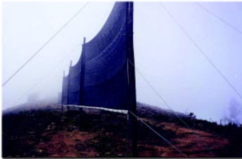
Fog-trapping nets capture moisture from the air
