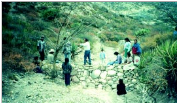
Building stonework systems to harness water
