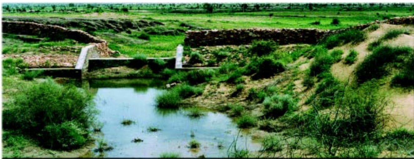
Community water-harvesting through water dam construction
