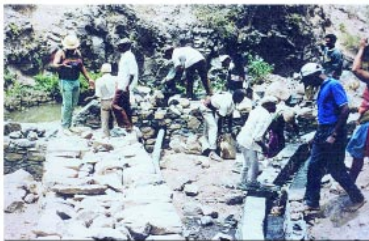
Community members build an irrigation channel
