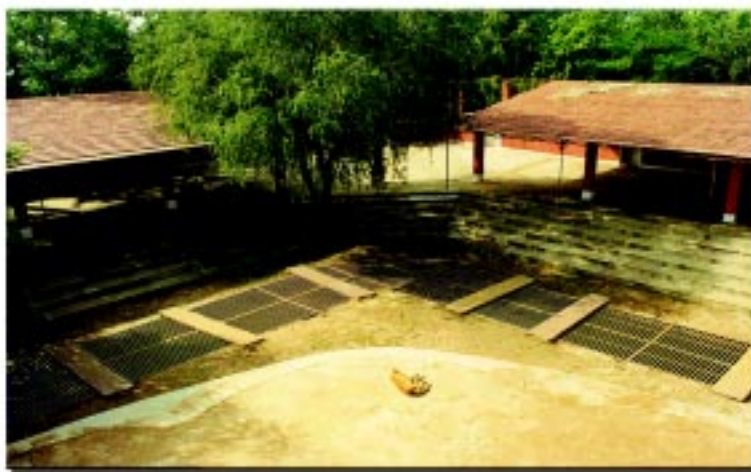
Underground water storage at the SWRC compound
