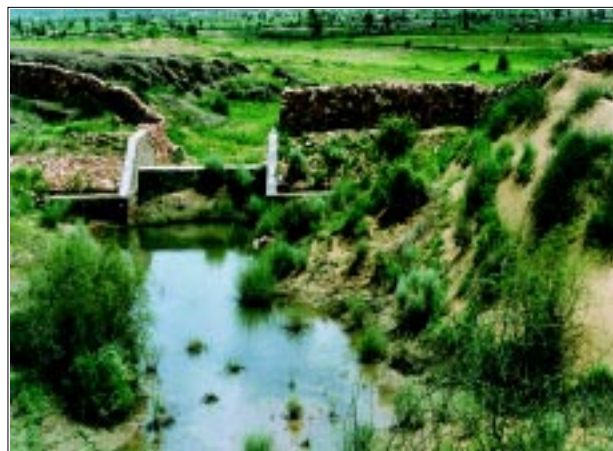
Community water dam
