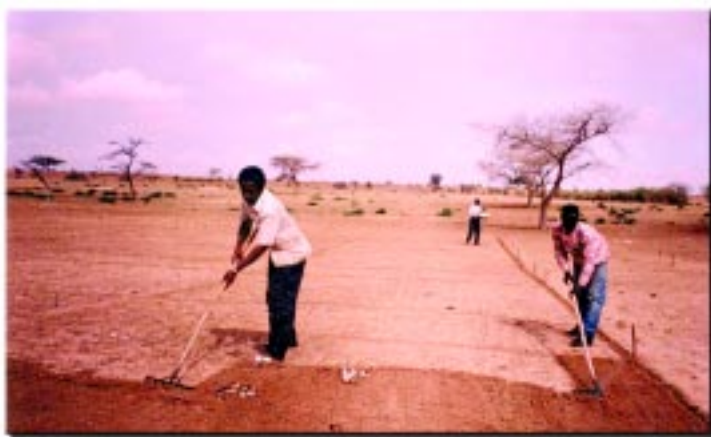
Clearing ground for school construction
