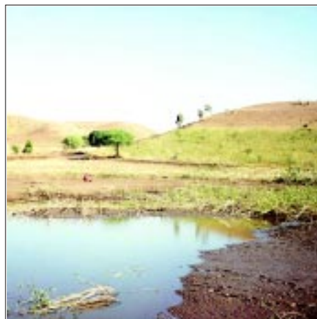
Water collecting dam
