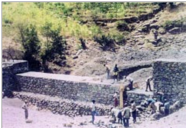
Construction of a major flood control dam and valley bank protection walls
