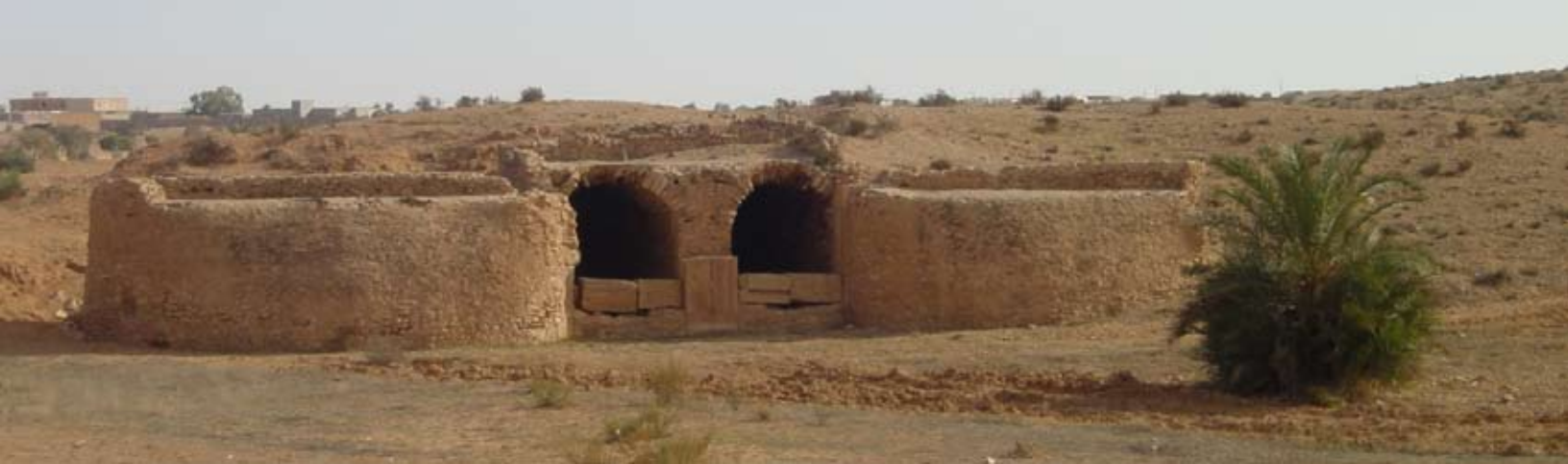
Photo: Ancient water storage system in Tunisia. Photographer: Boshra Salem
