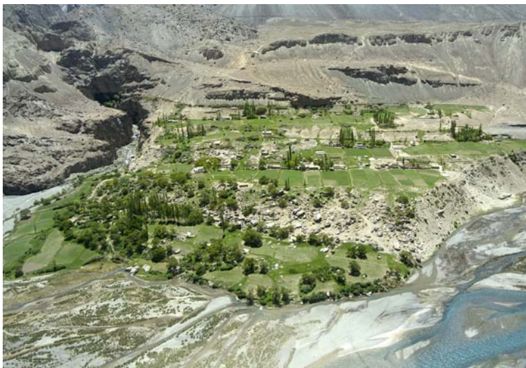
Plate 2: Aerial view of Barchidev village, Gorno-Badakhshan Autonomous Oblast. In much of GBAO the area available for irrigated agriculture is tiny whilst rainfall is too low and slopes too steep for rainfed agriculture. Such villages are also prone to natural disasters such as landslides. Photograph © Aga Khan Foundation/Jean-Luc Ray
