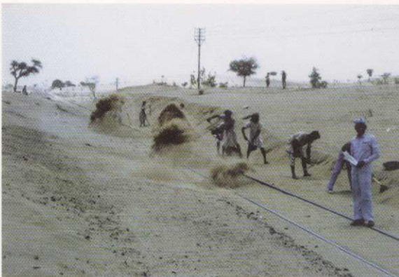
Photo 4-2-3 Sand movements affects infrastructure such as railways due to aerodynamic process (Barmer, India)
