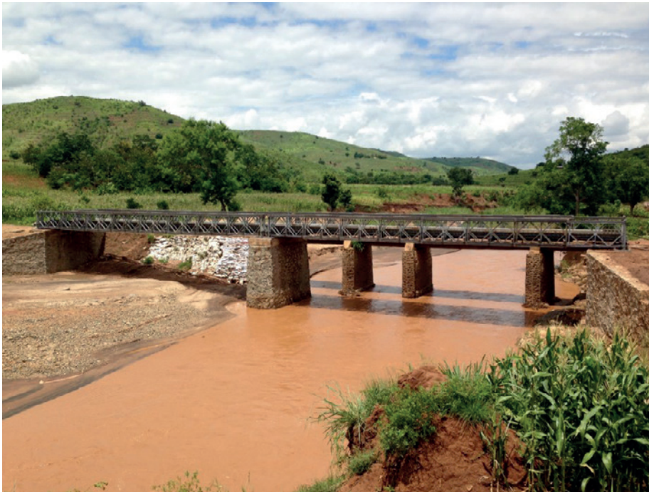
Newly constructed Bailey Bridge over Msuwazi River in Thyolo District, Malawi. Source: WFP
