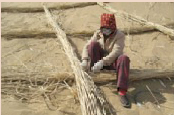
Initial stabilization of sand dunes using checkerboards
