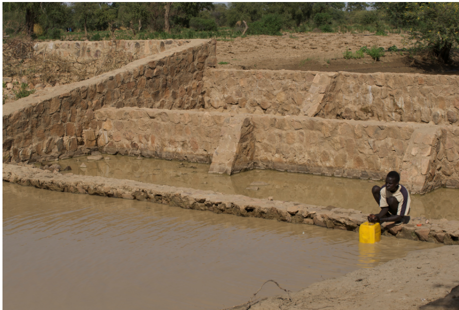
Figure 3: Example of a water spreading weir. Photo: © GIZ/Klaus Wohlmann
