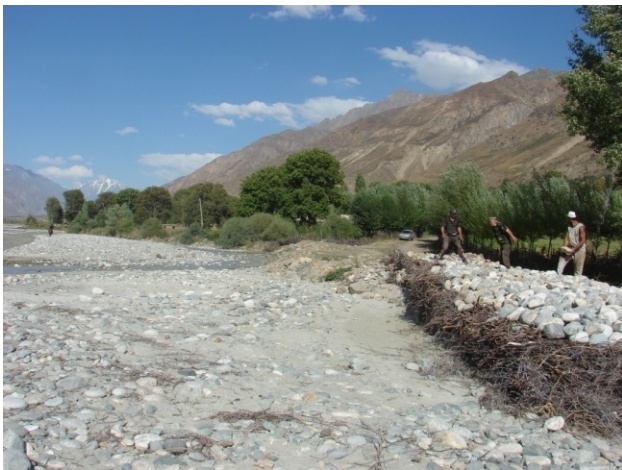
Figure 11: River bank protection
