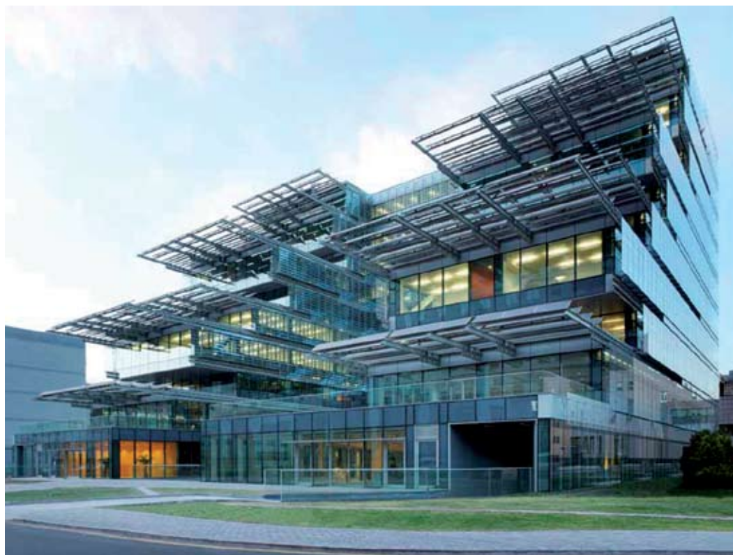
Sino-Italian ecological and energy-efficient building at Tsinghua University, Beijing
