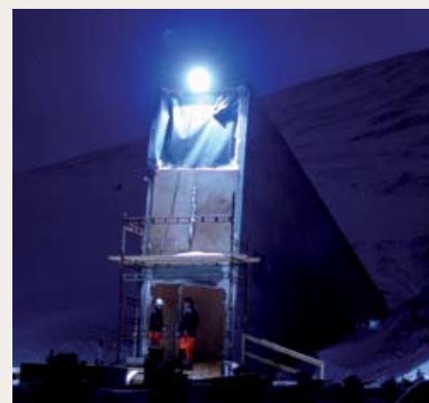
Construction workers stand beneath scaffolding at the entrance to the Svalbard Global Seed Vault.
