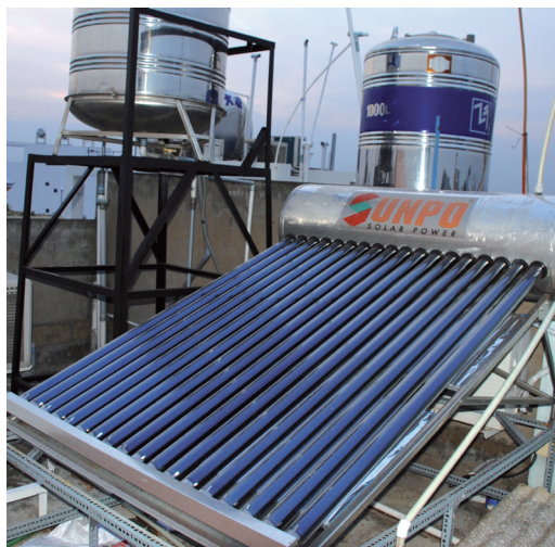
Solar water heaters are getting popular in Ho Chi Minh City, Vietnam. The Vietnamese government set up a programme in 2008 that subsidizes part of the installation costs of solar water heaters, supporting local manufacturers as well as saving 57 million kWh or 4 900 tonnes of oil equivalent per year.
