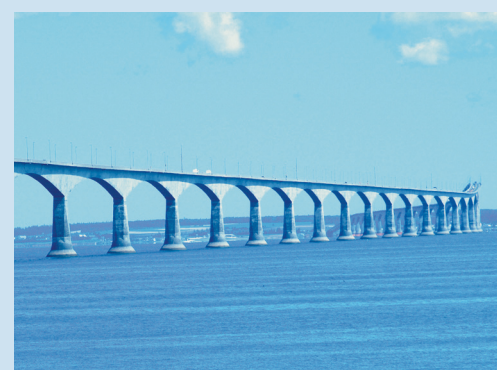
Source: Strait Crossing Bridge Ltd.
