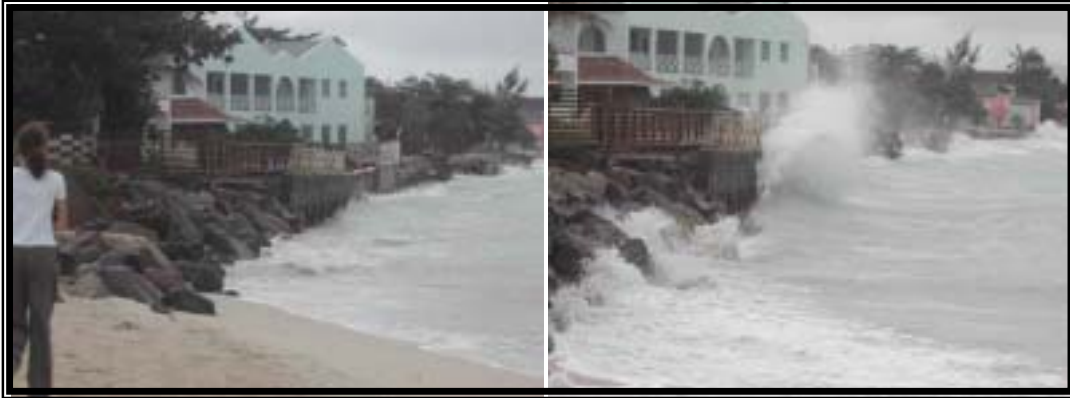
Figure 4.1: Pictures from Northwest Coast of Antigua demonstrating coastal erosion. Source: Environment Division Database
