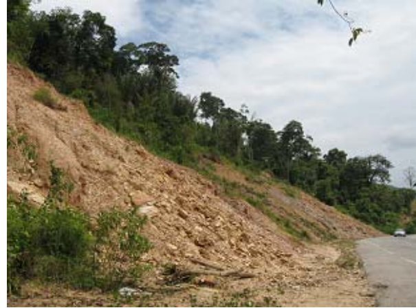
Landslide on North Coast Road, Trinidad
