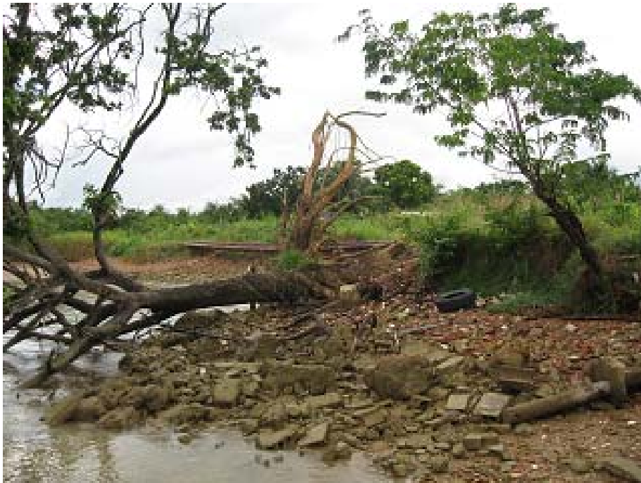
Photograph 4: Coastal erosion has become a common occurrence along Trinidad's southwest coast
