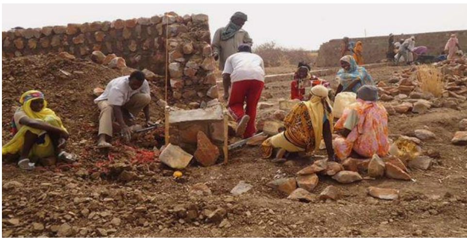
Community members volunteered to rehabilitate the Eware water retention structure
