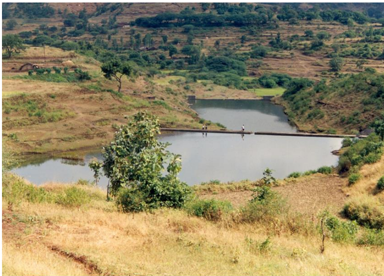
Water Harvesting Structures – A series of Check Dams
