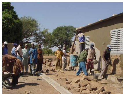
Construction by residents
