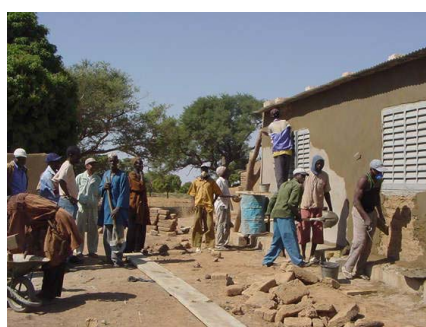
Construction by residents
