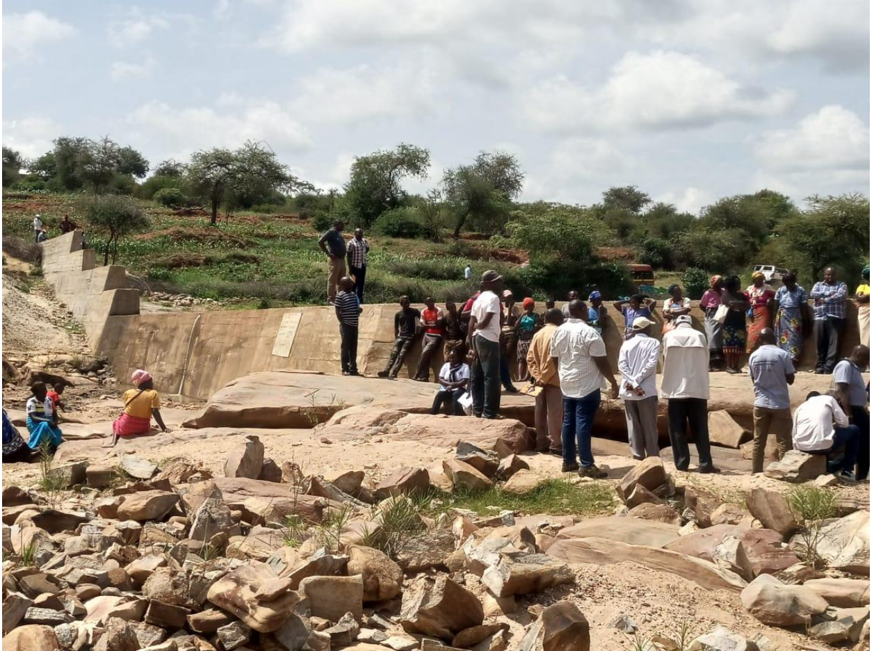
Plate 3: Launching the construction of Mwanja Sand dam in Mwingi subcounty, Kitui
